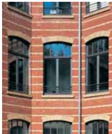
Hoch wärmegeädmmte Renovierung alter Bausubstanz in klarer Stahloptik High insulation renovation of old building structures with a clean steel look
